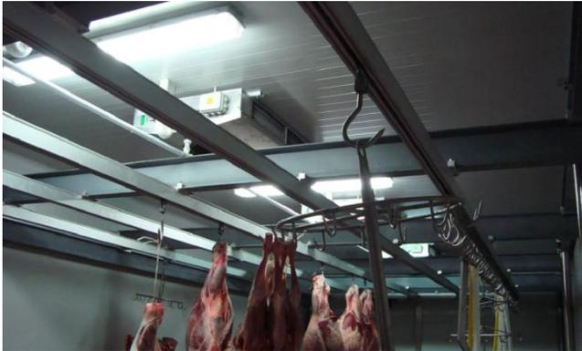
Figure 2 Evaporators location inside cold room n. ° 1.
